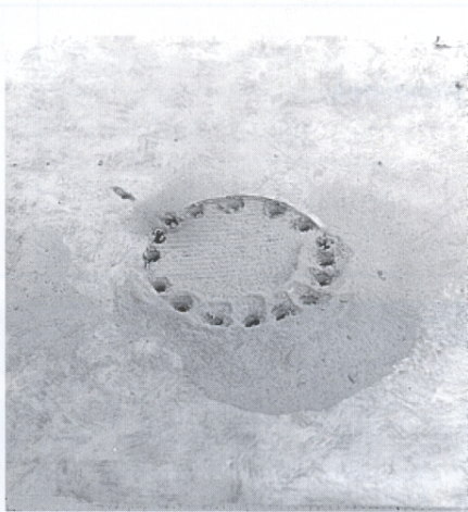
Drilled holes in slab
