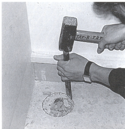
Chiseling of the hole
