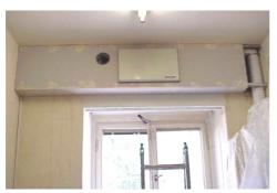
Casing of pipes made of gypsum plasterboard. An outlet into the kitchen will be provided with air diffuser.
