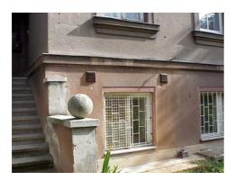
Front view of the basement flat. On the left side of the kitchen window there is an inlet for the ventilation unit and on the right side of the window there is an outlet from the cooker hood.
