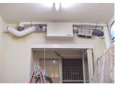
Ventilation unit above the kitchen window with the heater for preheating of the outdoor air on the right side. On the left side the distribution pipe continues through the partition wall to the living room. The rectangular pipe above the unit is an exhaust pipe from the cooker hood.
