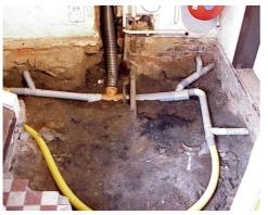
Chase excavated in the entrance hall served for drilling of perforated tubes into the sub-floor layers under the adjacent rooms. Horizontal PVC-U pipe connects the drilled tubes to the vertical exhaust from flexible rustless pipe, which is inserted into a free flue.
