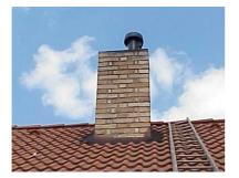
Vertical exhaust pipe ends with a roof fan above the chimney.
