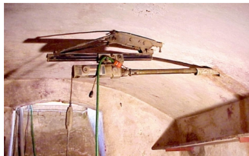
Drilling of perforated tubes from the cellar into the sub-floor region
