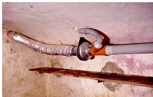
All drilled tubes are connected with a PVC-U exhaust pipe to a fan. A silencer is mounted between the fan and the outlet.
